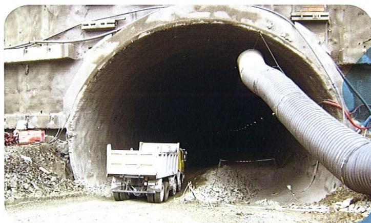
Our ventilation duct situated in the tunnel
